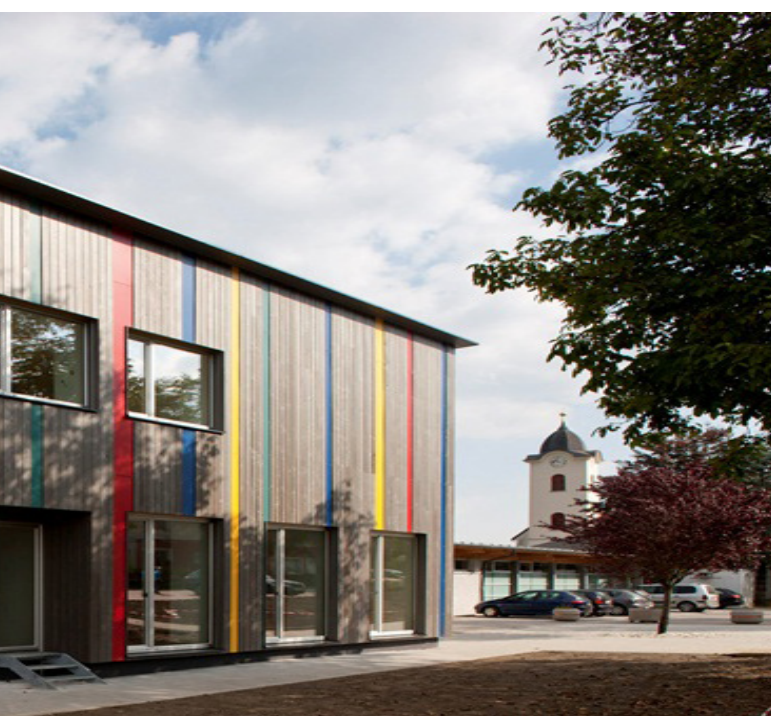
Picture 1 St. Leonard before retrofit
